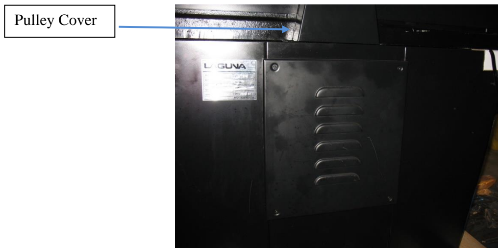
FIGURE 14: Pulley Cover installed
